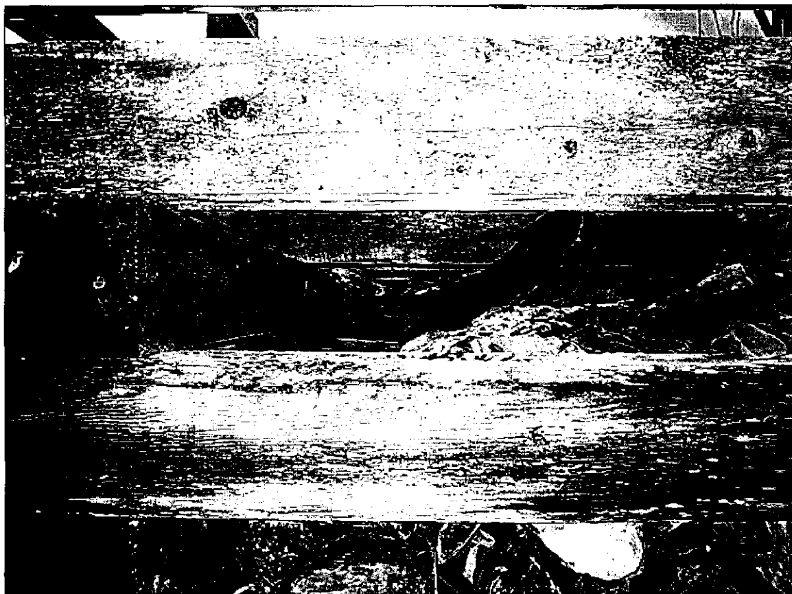
Ballast missing from crib work
